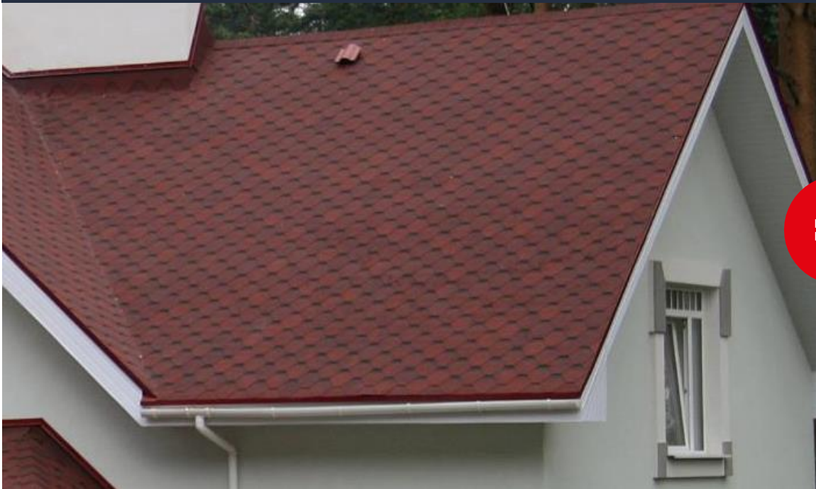
The roof with single-layer roofing shingles
