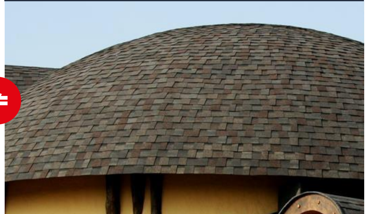
The roof with multilayer roofing shingles
