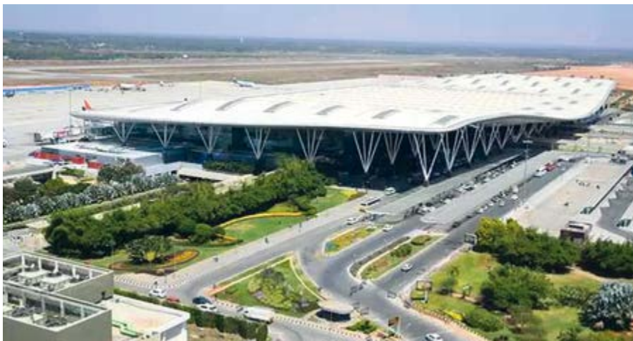
Bengaluru, India BANGALORE INTERNATIONAL AIRPORT - TERMINAL 2
