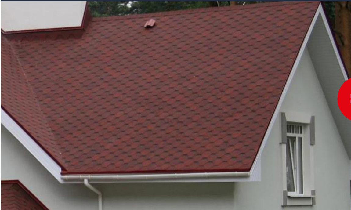
The roof with single-layer roofing shingles
