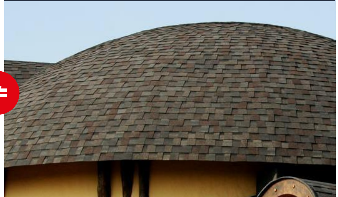
The roof with multilayer roofing shingles
