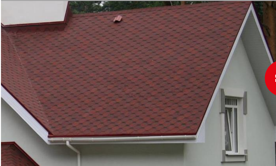
The roof with single-layer roofing shingles
