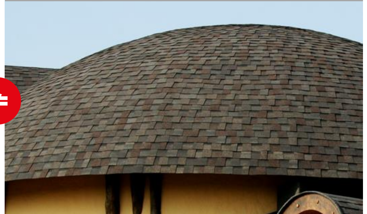
The roof with multilayer roofing shingles
