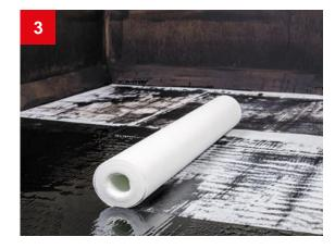
Install reinforcement layers of a fiberglass between all the layers of mastic.
