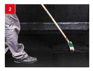
Apply 3 layers of a roofing mastic (3-4 mm) by pouring and levelling over the surface with a squeegee or a brush.
