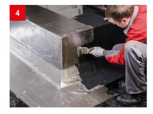
The resulting monolithic layer must be protected from the impacts of UV and temperatures.
