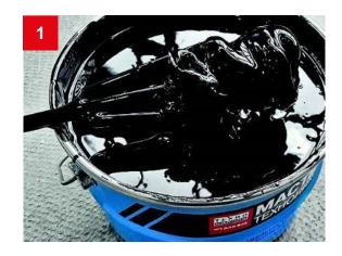
Carefully mix the primer by a lowspeed drill with the special nozzle.
