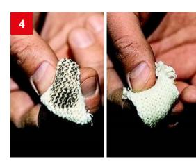
Allow the treated surface to stand until the full drying of the primer. It is possible to check whether the primer has dried by pressing a dabber to it: there should be no bitumen traces on the dabber pressed to the dried primer.
