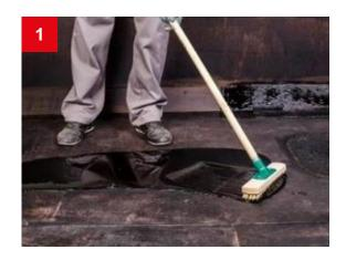
Apply the first layer of mastic on the primed surface.
