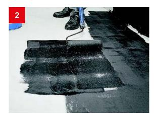
Apply the primer manually onto the cleaned surface with brushes, sweepers or paint rollers.
