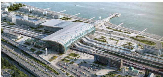
Adler Railway Station Adler, Russia
