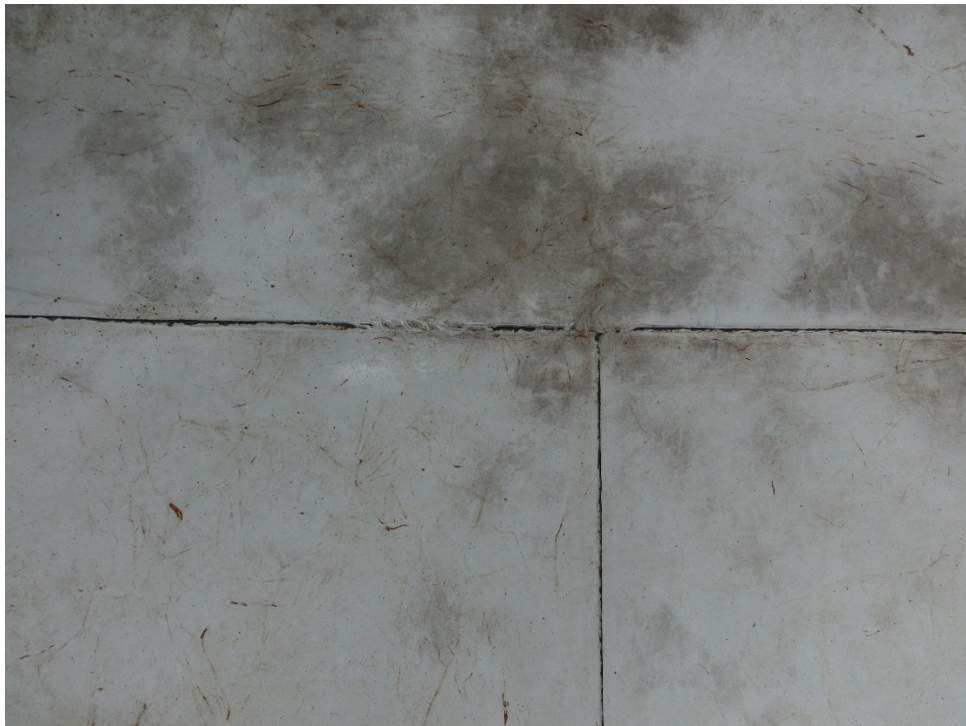
Fig. 3: T-joint at the end of the test
