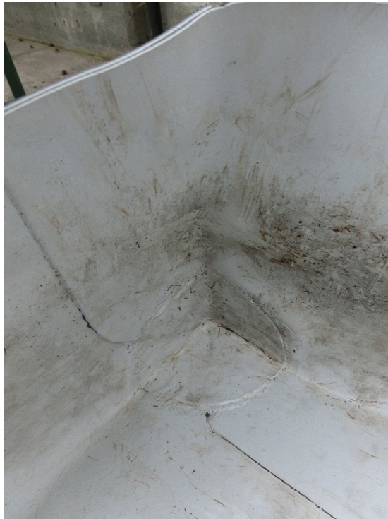
Fig. 2: Corner of the test specimen at the end of the test
