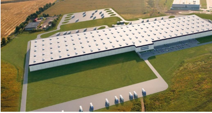
Distribution centre Tchibo, Cheb, Czech Republic LOGICROOF V-RP 1.5 mm | 65 000 m 2
