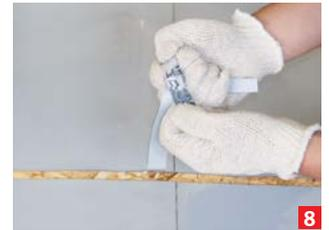
5. Corners of membranes should be cut with scissors to the round shape. It is recommended to avoid creating multiple cross overlaps of more than three sheets.
