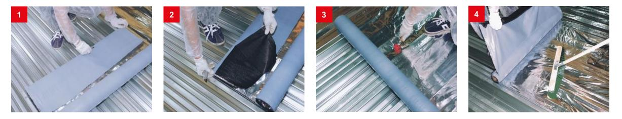
Cut the siliconized anti-adhesion film at the distance of 30-40 cm from the beginning of the roll by means of roofing knife.
