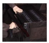
In this case, one should cut the material into shorter segments and first install the material on the lower part of the foundation on its' entire perimeter.
