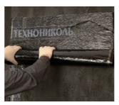
At first, carefully cut and remove the protective film in 10-15 cm from the beginning of the roll and attach the material at the top. Then install the main part of the roll by gradual removing the protective film, unrolling the membrane and smoothing it on the surface.
