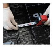
The longitudinal overlap should be minimum 100 mm, transversal - not less than 150 mm. Transversal overlaps of adjacent rows should be displaced for at least 500 mm.
