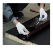
Start installing the first row of the membrane. Carefully cut and remove the protective film in 10-15 cm from the beginning of the roll.
