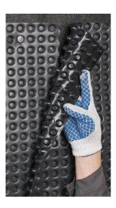
The lateral overlapping of adjacent rolls should make at least **4 studs**.
