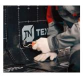
For better adhesion, clean the overlap zone from dirt and dust with the clean and dry cloth just before the formation of transversal or longitudinal overlap and press it with the roller after the installation of the material.
