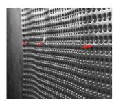
Pierce through the roll of profiled membrane with the tip of the fixture.
