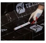
The longitudinal overlaps should be minimum **100 mm**.
