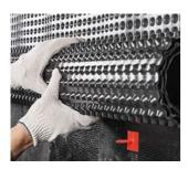
Unwind smoothly the roll of profiled membrane fixed at the basement level in downward direction.
