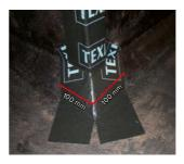
The reinforcement of the external corner is performed in two steps. At first, one should reinforce the lower part of the corner adjacent to the horizontal surface. For this, make a patch from the main waterproofing membrane with special cutouts so that the element can be installed without waves and folds. The element should overlap both sides from the corner axis for **100 mm**.
