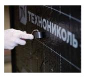
Always use the silicone roller to ensure reliable adhesion of the material to the surface and avoid the formation of air bubbles and creases, which can worsen the waterproofing properties.
